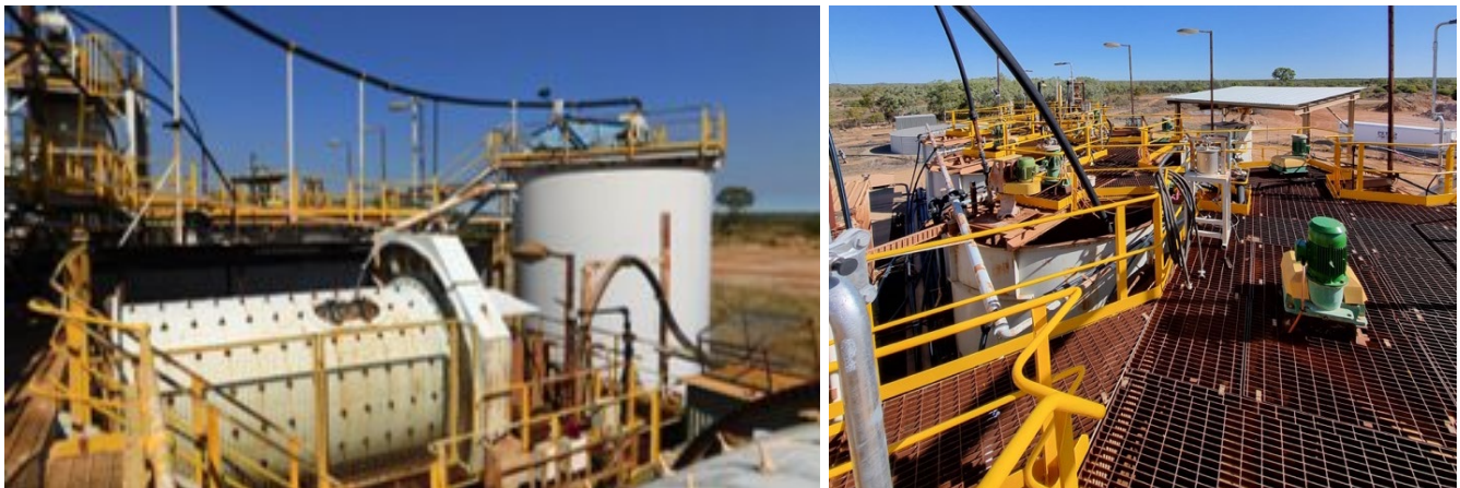
Figure 3 Georgetown Gold Processing Plant
